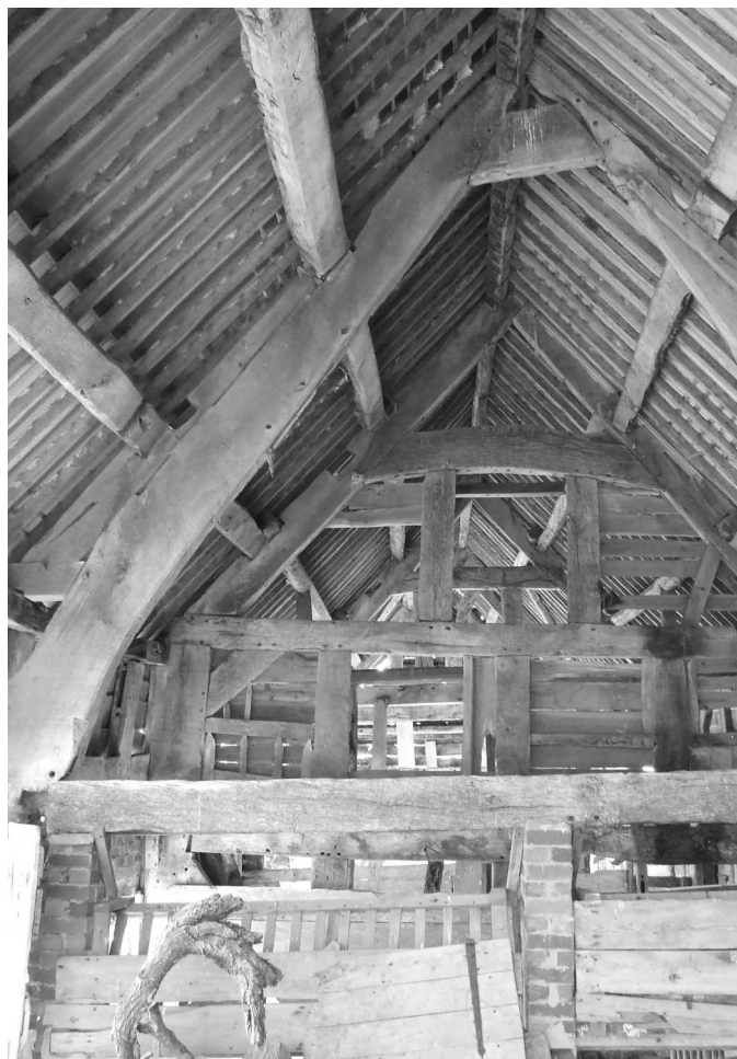
Figure 6: The barn at Ffynnant, with the cruck-framed unit, originally a dwelling, in the foreground, and the later box-framed extension behind.
