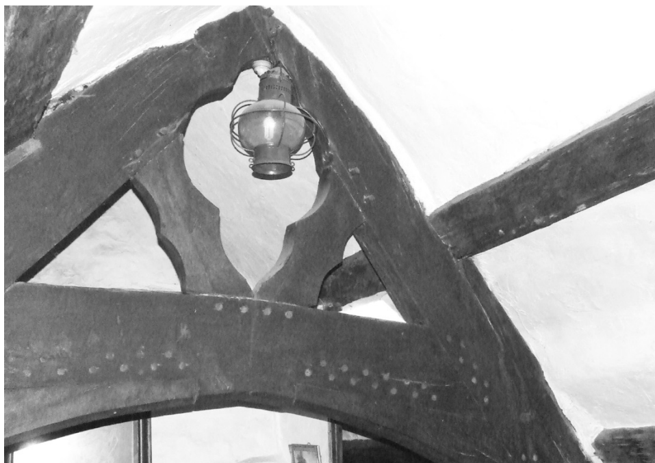
Figure 2: Cusped bracing and fine carpentry at Hafod Ysbyty.
