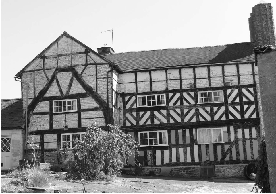
Figure 5: Ffynnant farmhouse, showing the cruck-framed unit on the left with a later heightened roofline, and the later box-framed extension to the right.
